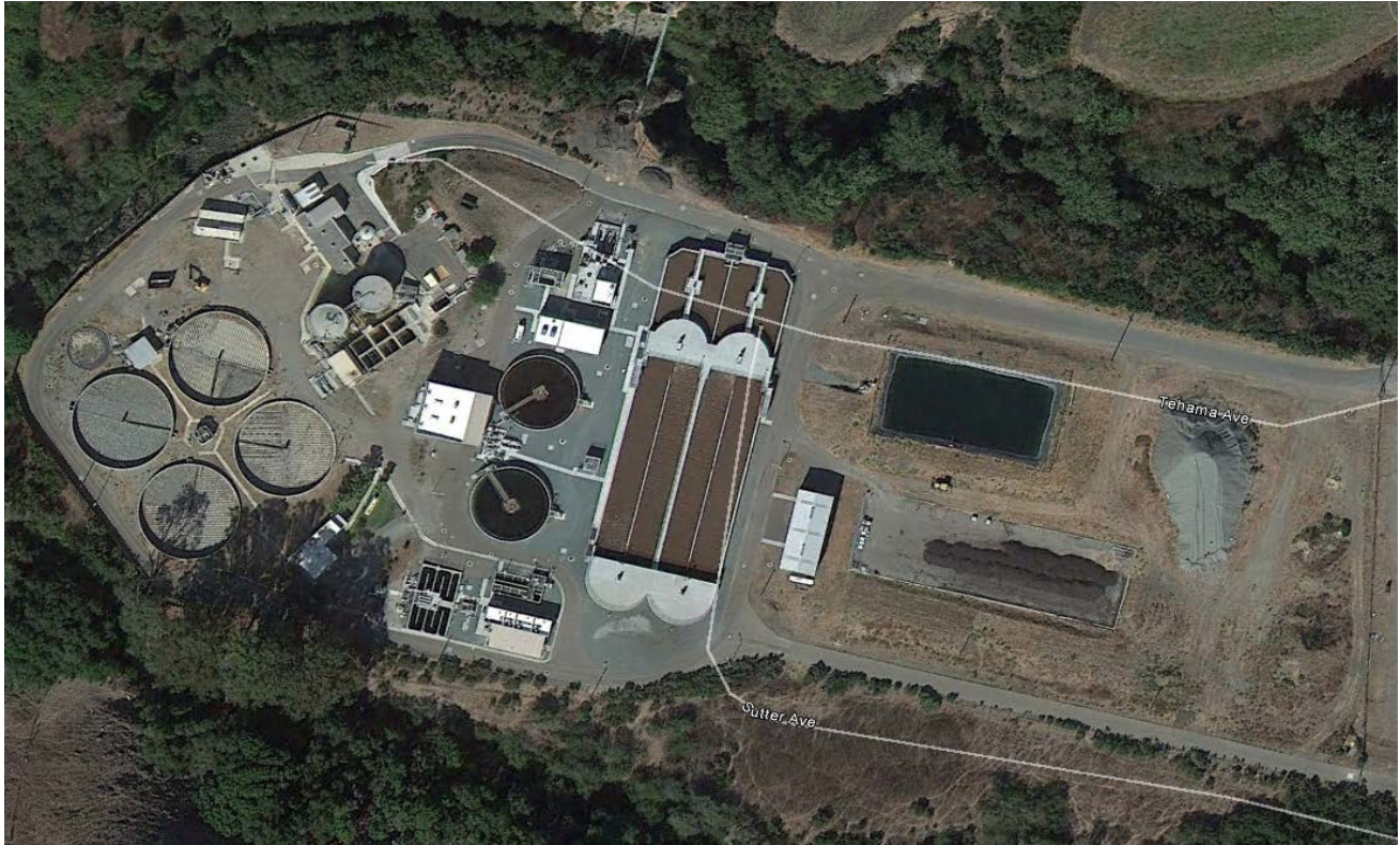
Figure 8. CMC WWTP aerial photo
